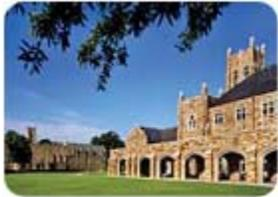
*The exterior walls of the library are built from solid pieces of rubble stone, while Indiana limestone and Vermont slate were used for architectural details such as arches and window surrounds.*
