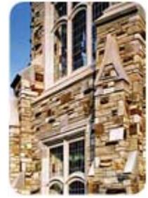
*The rubble stone pieces were intentionally laid in a random pattern, and consideration was also given to the varying color of the stone during the installation process.*
